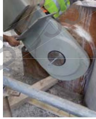
Figure 28. Out-rigger Hinge Connection 28/05/2013 *
